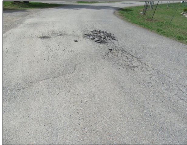
Picture 2 – Fatigue and Block Cracking (3 rd Street)
