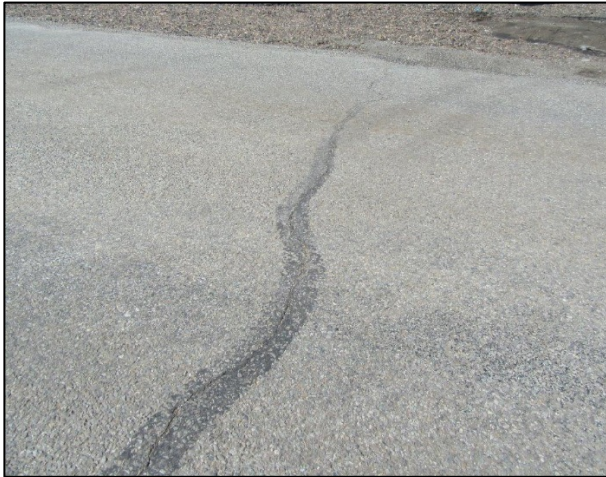
Picture 1 – Transverse Cracking (1st Street)
