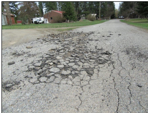
Picture 3 – Fatigue Cracking (Bennett Street)
